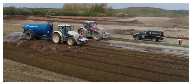
All works were tested during the construction process for MCV and CBR
